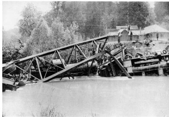
Collapse of steel bridge, Münchenstein (1888)
