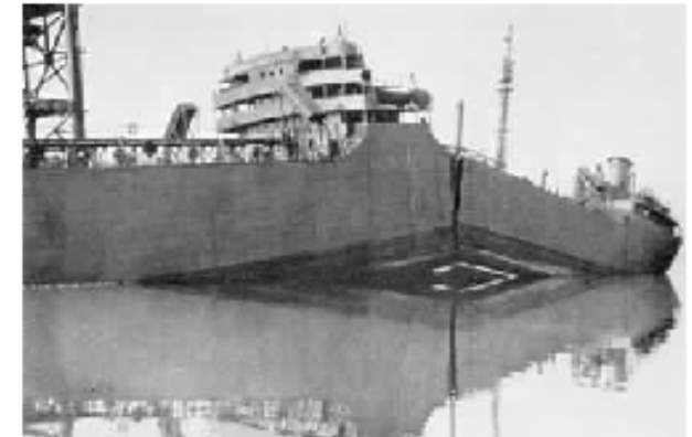
Brittle fracture of welded structures (Liberty ships (1940-45)
